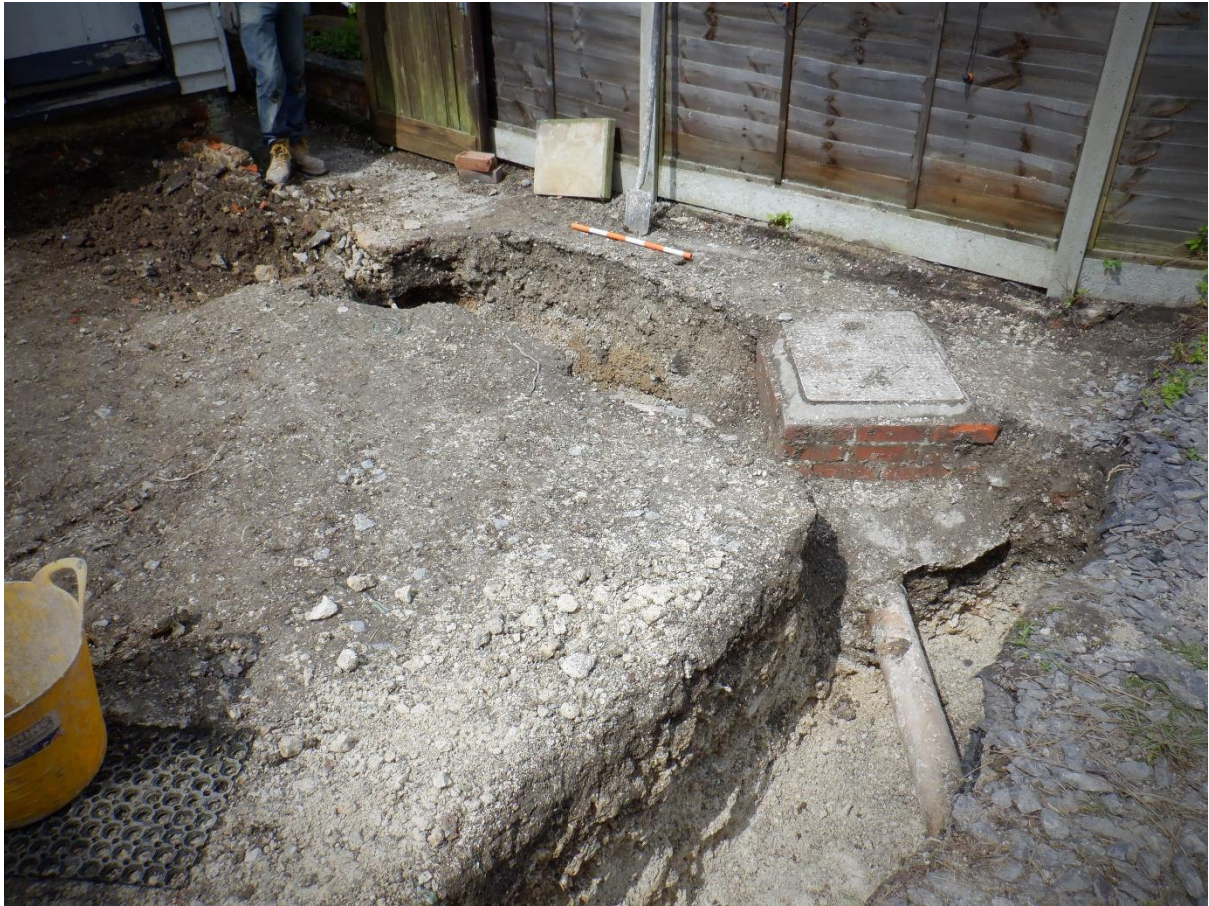
Plate 3. Ground reduction and trenching (looking NNW)
