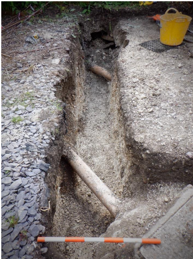
Plate 4. Foundation trenches (looking East)
