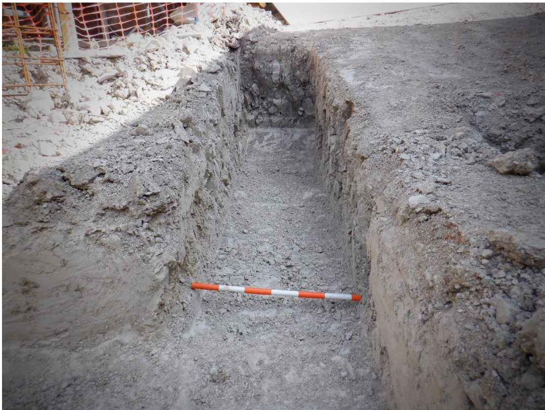
Plate 6. Foundation trenches (looking West)
